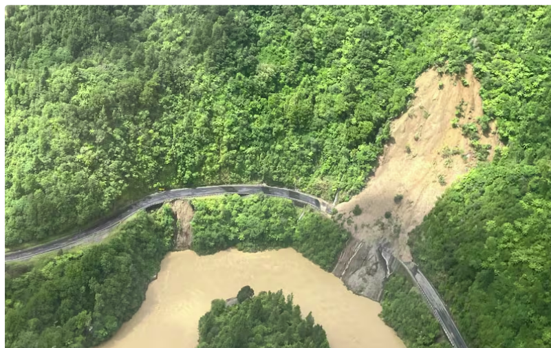
A slip blocks State Highway 2 in January. Photo: Supplied/NZTA
